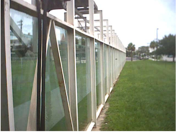
Florida Tech's Ocean Engineering wave channel for testing shallow water active and passive water surface imaging systems.
